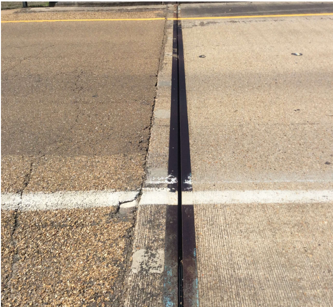
PHOTO 1 Description Joint material missing abutment 1
